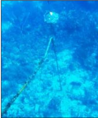
Example of an old chain and cement mooring with riser
